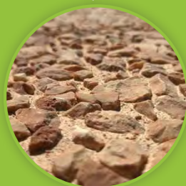
Examples of exposed aggregate concrete surfaces: Surface characteristics will also depend on choice of cement, aggregates, pigments ...
