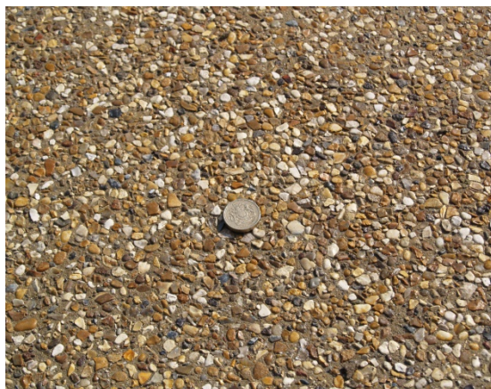
Pictures: Example of exposed aggregate concrete surface where Hebau CSE® deactivators were used. More details available on request.
