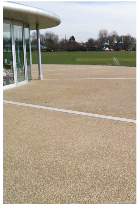
Pictures: Example of exposed aggregate concrete surface where Hebau CSE® deactivators were used. More details available on request.
