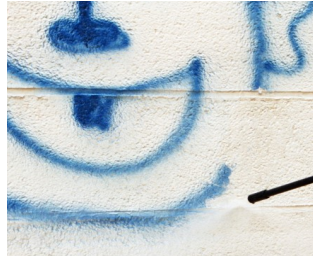
If the protected surface is soiled with graffiti: clean surface with a high pressure cleaner. Then re-apply the PROWALL II onto the cleaned areas.
