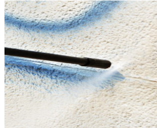
If the protected surface is soiled with graffiti: clean surface with a high pressure cleaner. Then re-apply the PROWALL II onto the cleaned areas.
