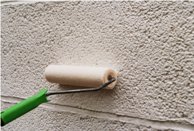
Application of PROWALL II , e.g. with a roller.
