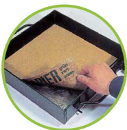
Lay the retarder paper in the mould (printed side down)
