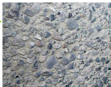
Close-up view of a construction joint surface which has been made with the help of a CSE® Deactivator
